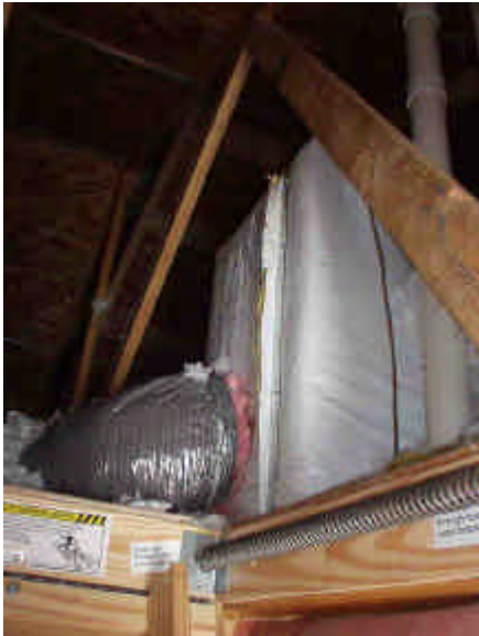
^^ The trunk/plenum/duct connection is a particularly critical joint for flex duct systems. Make sure that they are mechanically secured and sealed. >>
