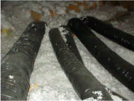
<< Two views of a leaky attic mounted return duct system. The left view is a panned interior partition wall top and the right is a set of duct/trunk connections. v v
