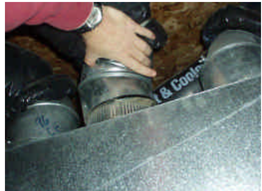
^^ The trunk/plenum/duct connection is a particularly critical joint for flex duct systems. Make sure that they are mechanically secured and sealed. >>
